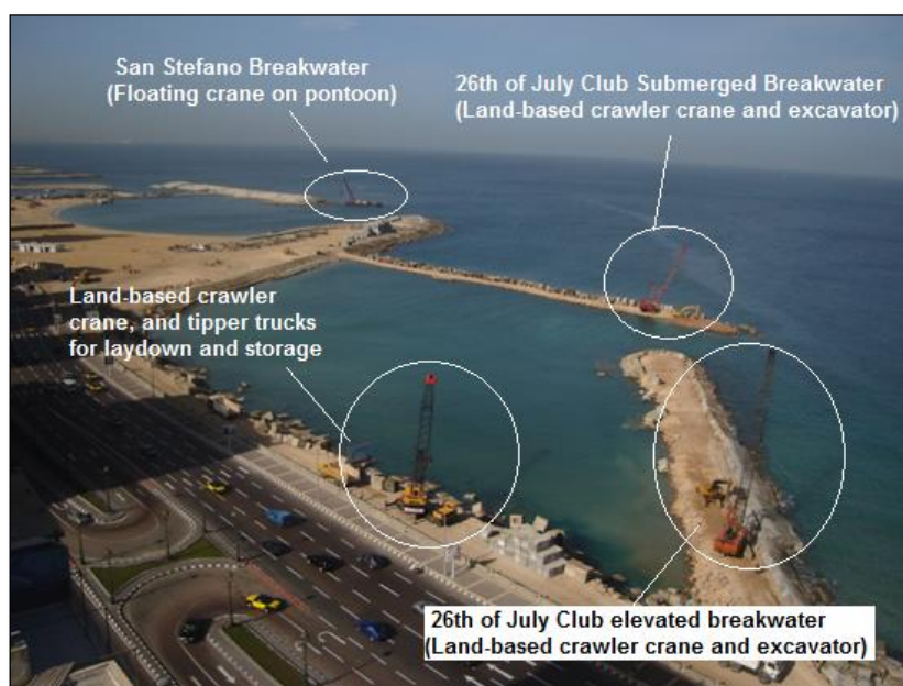
Figure 2-21: Combining land-based and waterborne equipment (Courtesy of AF Co.).
